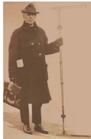
Mr. Will Damman with his invention, "The Toe/Camber Gauge" 1917
